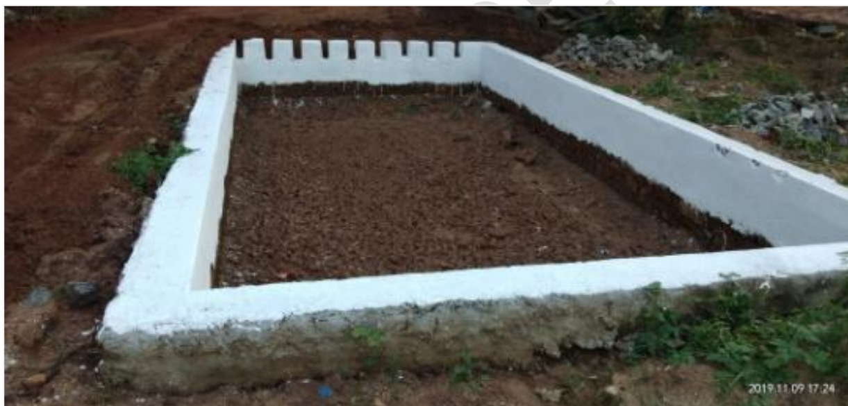
Plate 2: Rain water harvesting in the premises
